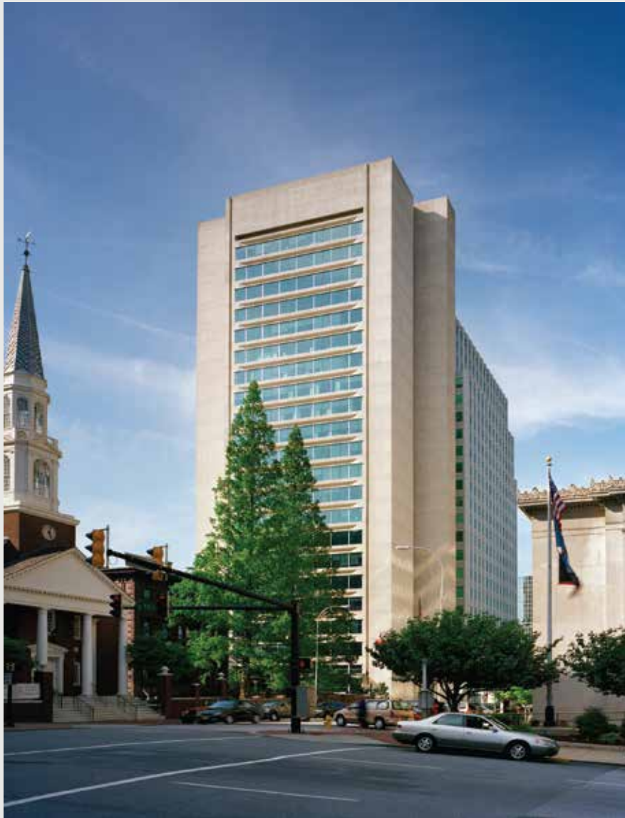
Exterior of 1105 N Market
